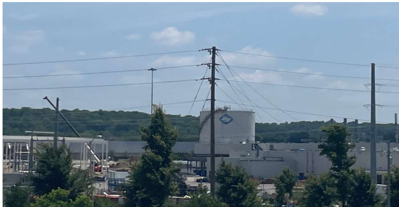
FIGURE 49: IMAGE OF FUYAO ADDITION UNDER CONSTRUCTION.
